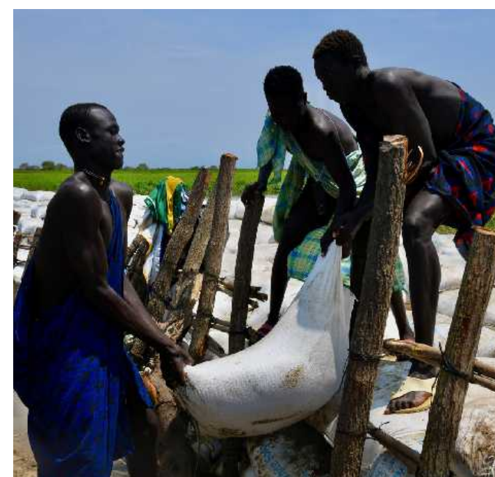
Communities in Bor South construct flood dyke to mitigate against the impact of extreme flooding. Photo © Joseph Basoga
