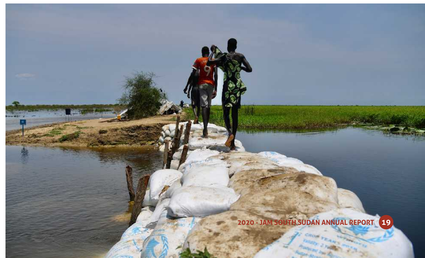
Communities in Bor South construct flood dyke to mitigate against the impact of extreme flooding. Photo © Joseph Basoga
